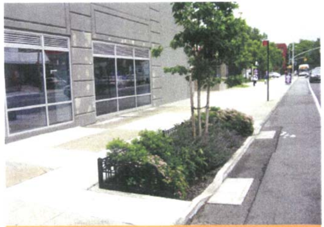
Bioswales use planted areas to reduce drainage
